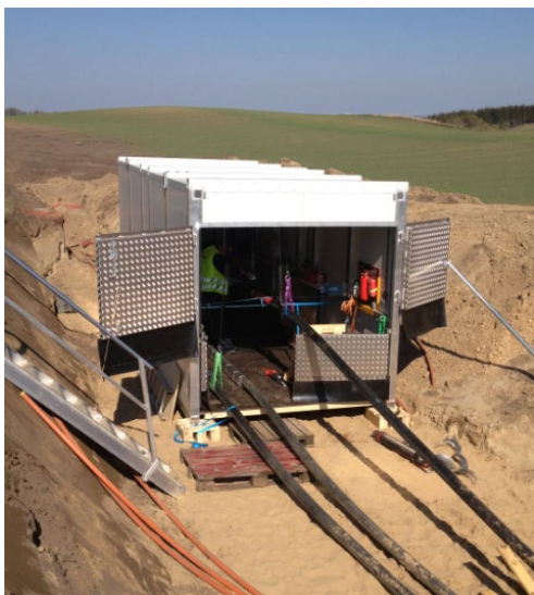
Figur 31 Montagecontainer placeret over en muffesamling.
